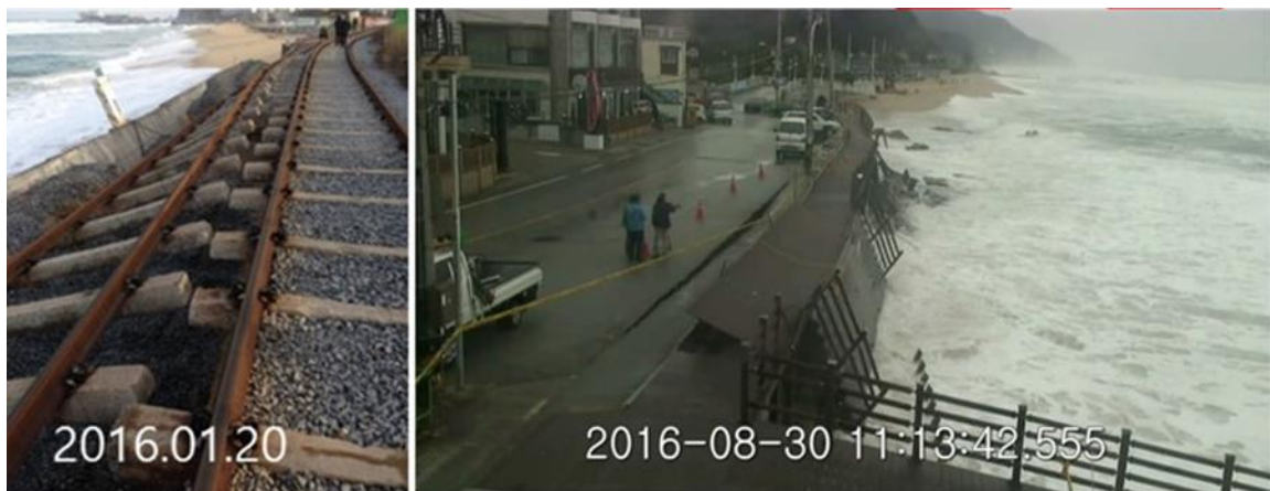
Figure 2. Structural damages in the northern (left) and southern (right) sides of the Jeongdongjin beach.
