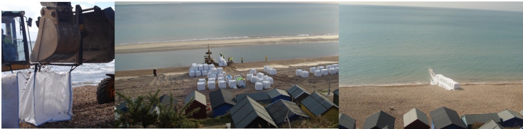
Figure 2. Left and centre: groyne construction, filling the geobags and deployment of the lower section of the structure during low tide the 27 th September 2007. Right: View of the temporary structure from the top of Hordle Cliff the 6 th October 2007.
