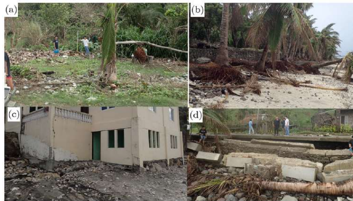
Figure 4. Pictures of: (a) debris lines; (b) exposed roots of coconut trees; (c) scour around a house; and (d) collapsed seawall
