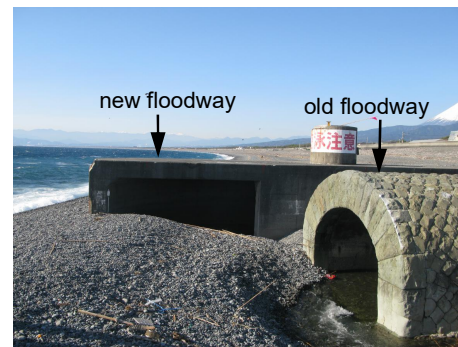
Figure 2. Horseshoe and rectangular mouths of old and new Shin-nakagawa floodways, respectively, and deposition of gravel in front of the mouths.
