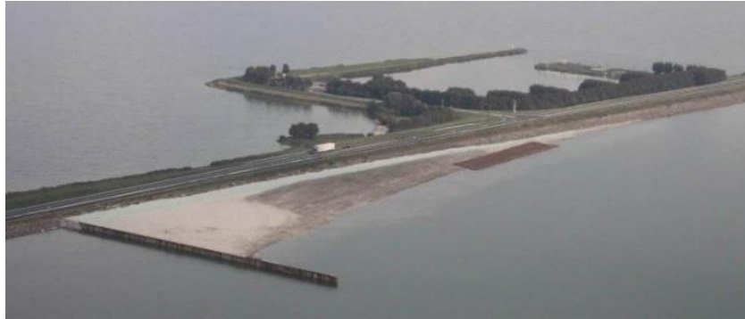
Figure 1 Overview of pilot section direct after construction in September 2014 showing the sheet pile wall and the plot in which clay is mixed in the top layer of the sandy test section (photo: Mennobart van Eerden).
