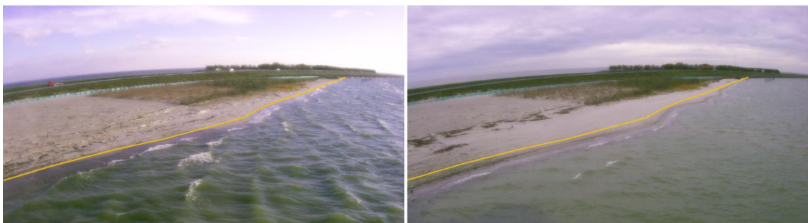
Figure 6a View on the pilot section on November 19 before the storm; Figure 6b View on November 21 after the autumn storm. The yellow line indicates the pre-storm position of the waterline on November 19, 2016.
