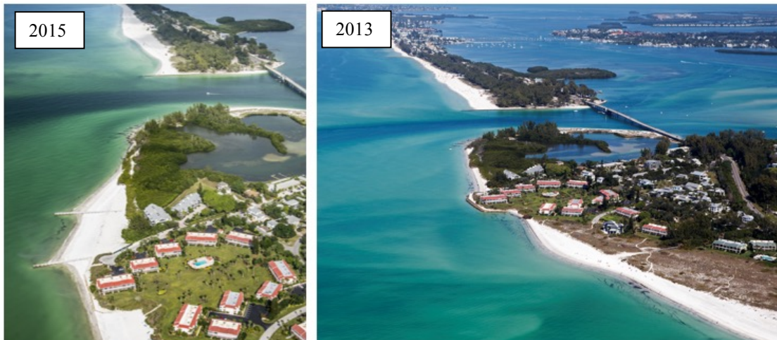
Figure 10. Recent conditions and erosion control structures to address chronic beach erosion along the sand spit at the north end of Longboat Key
