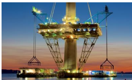
Figure 1: Queensferry crossing under construction
