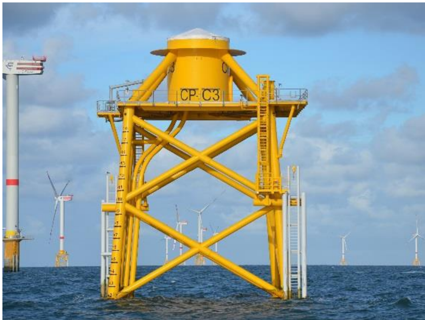
Figure 2: Jacket foundation (centre) and monopile foundation (left) on the C-Power OWF.
